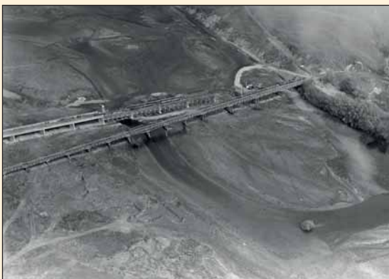
Red Bridge built 1950
