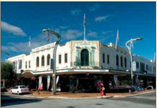
Hastings i SITE, Visitor Information Centre
