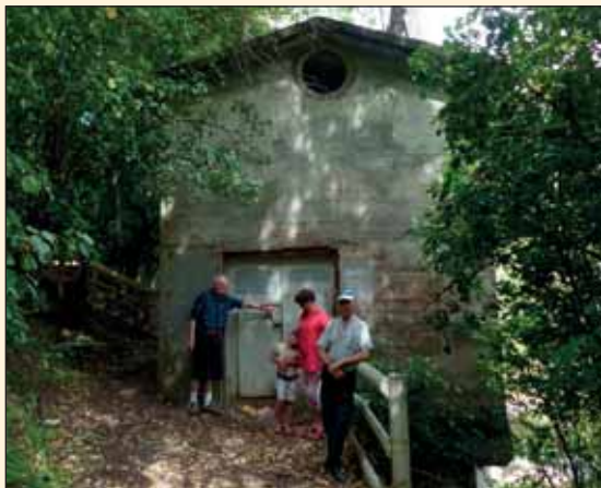
Old Turbine House & Surge Chamber, Maraetotara - Ivan Hughes
