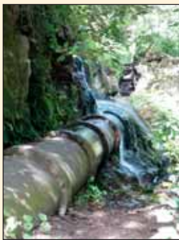
Old Penstock Pipes, Maraetotara Ivan Hughes
