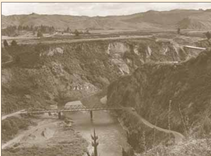
Mohaka River bridges – the old and the new - Looking downstream
